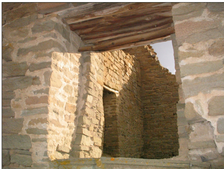
Juniper door lintels at Aztec Ruins in northwestern New Mexico.
